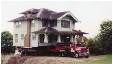
MN Rules, Chapter 1300.0220 Subp. 4 Moved buildings: Buildings or structures moved into or within a jurisdiction **shall comply with the provisions of the code for new buildings or structures**. Exception: A. Buildings designed to comply with Chapter 1311: or B. A residential building relocated within or into a municipality need not comply with the Minnesota Energy Code or Minnesota Statutes, 3268 430
